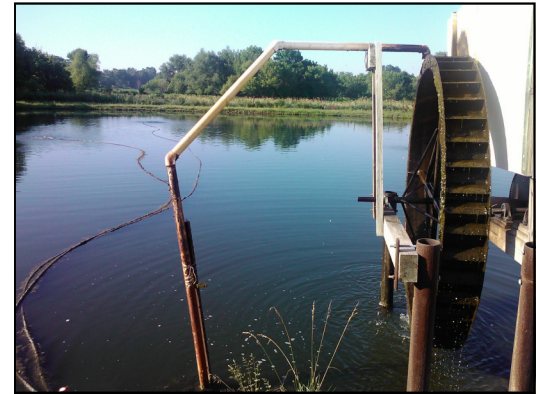
Spring-powered aeration system
